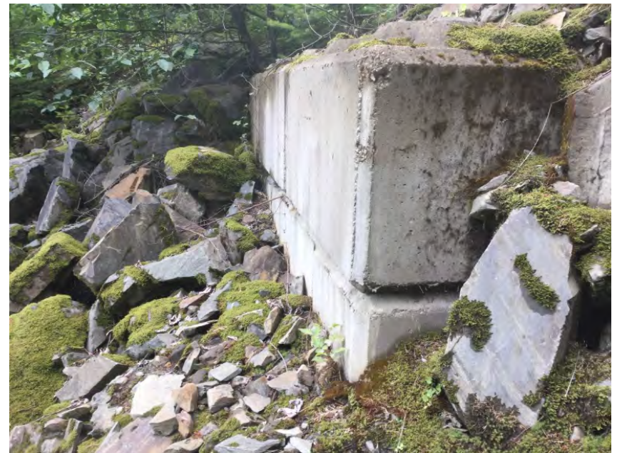
Downstream right abutment wingwall
