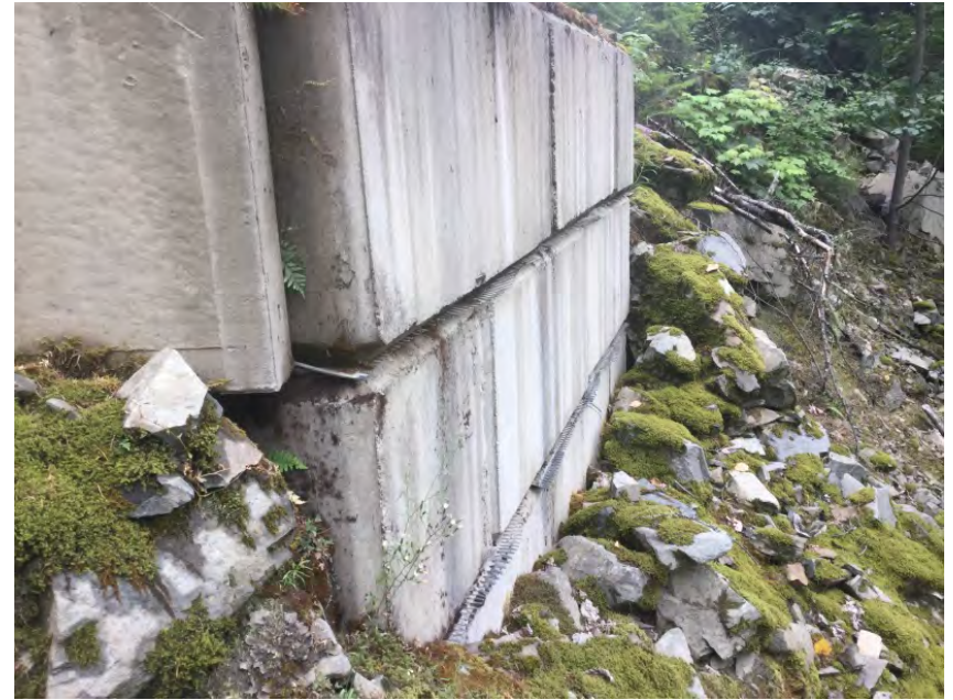
Downstream left abutment wingwall
