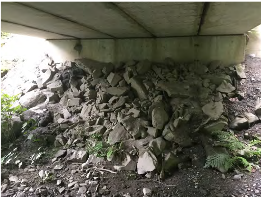
Right Bank Abutment when facing downstream
