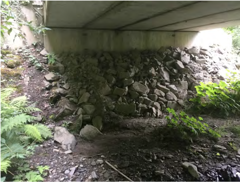
Left Bank Abutment when facing downstream
